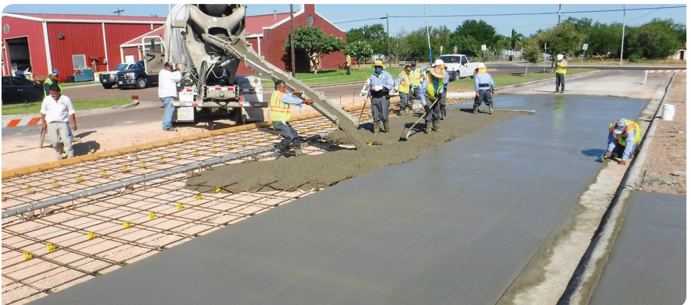
Construction is underway at Southside Park, the City's newest recreational facility.
