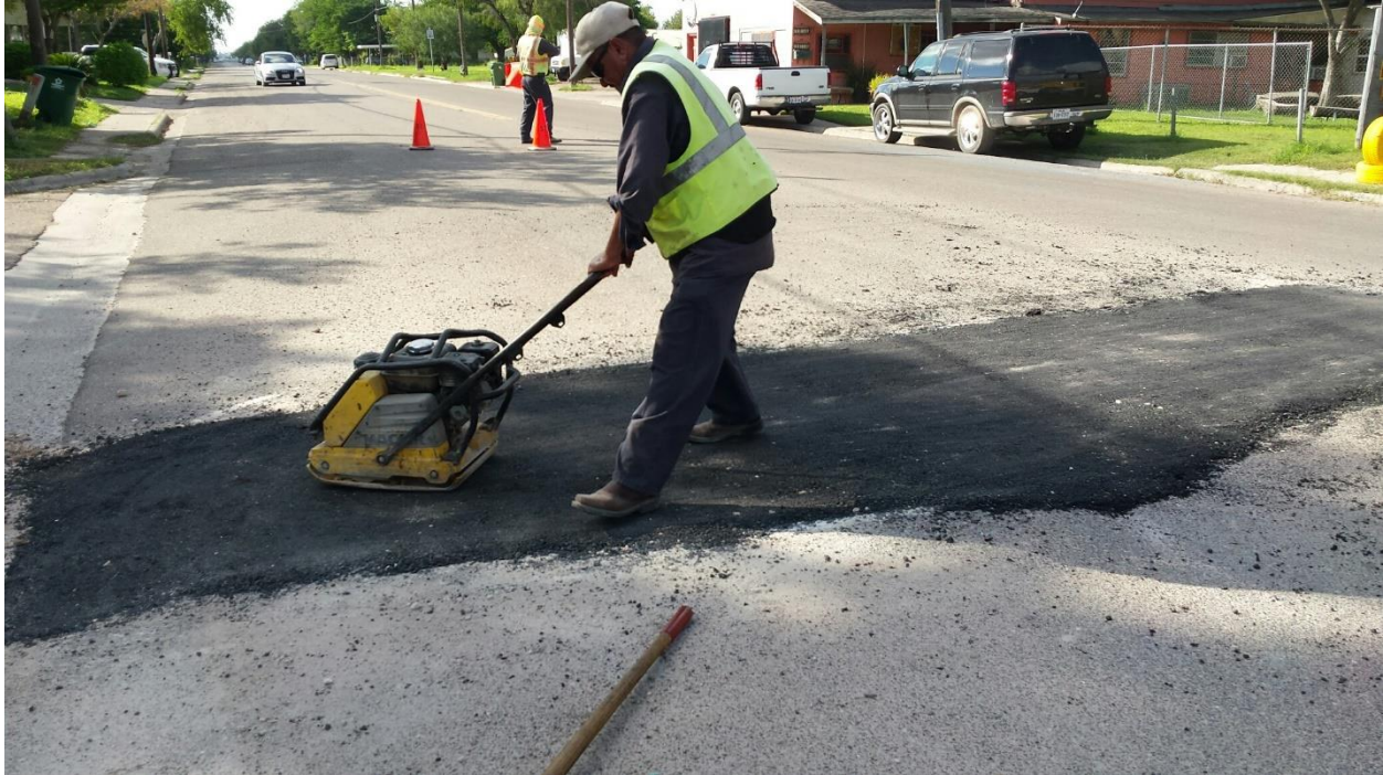
Street Maintenance Crew patching big potholes with the extra Hot Mix.
