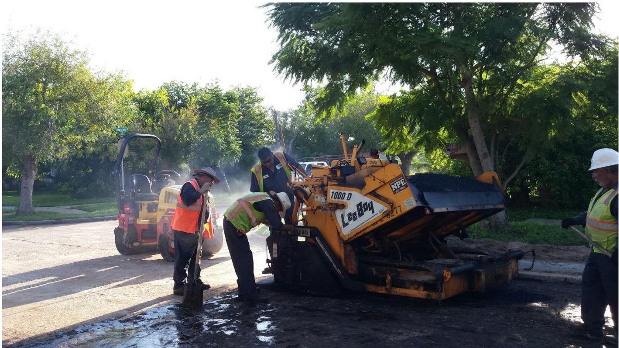
Street Maintenance Crew pouring TAC Oil in preparation of paving S. Travis Street.
