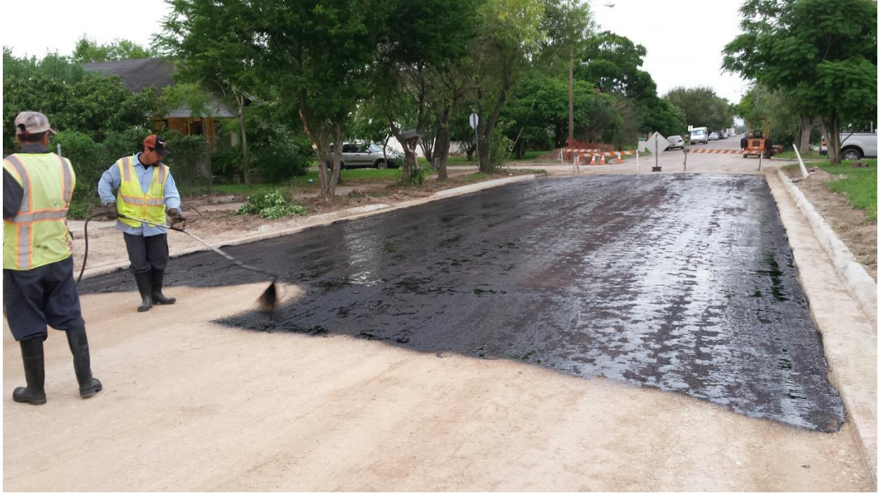
Street Maintenance Crew pouring TAC Oil in preparation of paving S. Travis Street.
