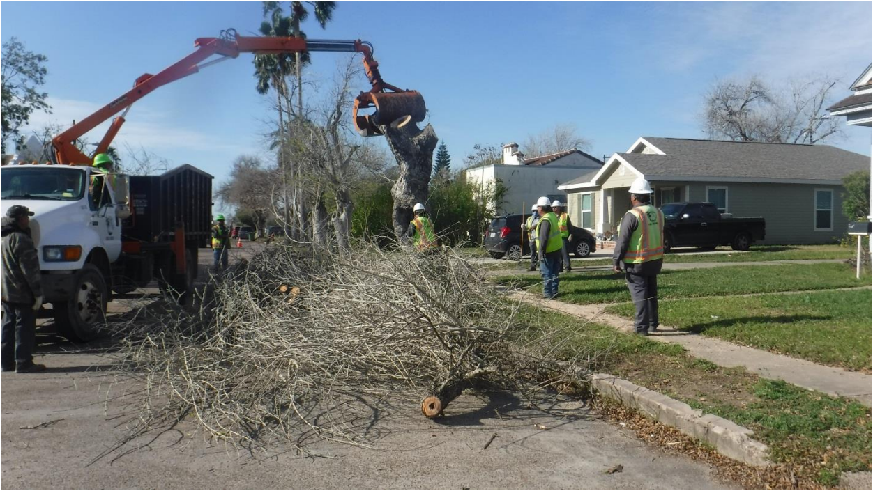
Public works ground crew cutting down old and hollow trees hosting potential danger.
