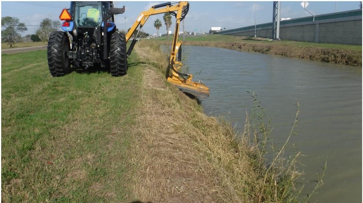
Public Works ground crew maintaining grass along Resaca banks.
